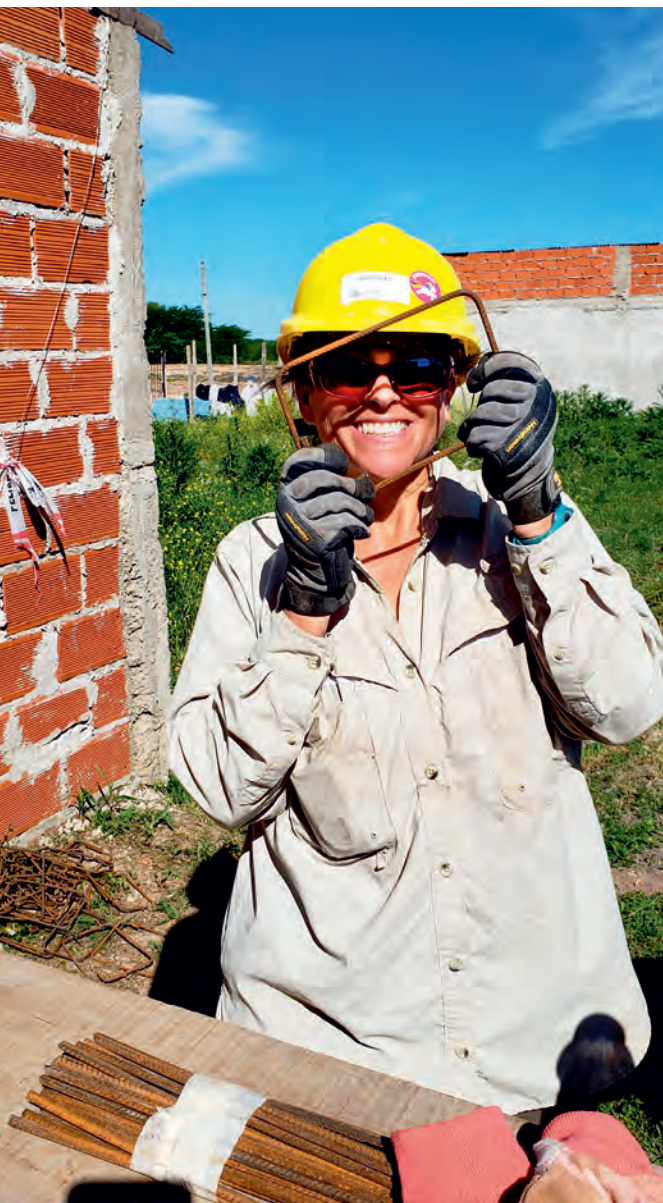
Bending rebar for a home in Buenos Aires, Argentina with Habitat.
